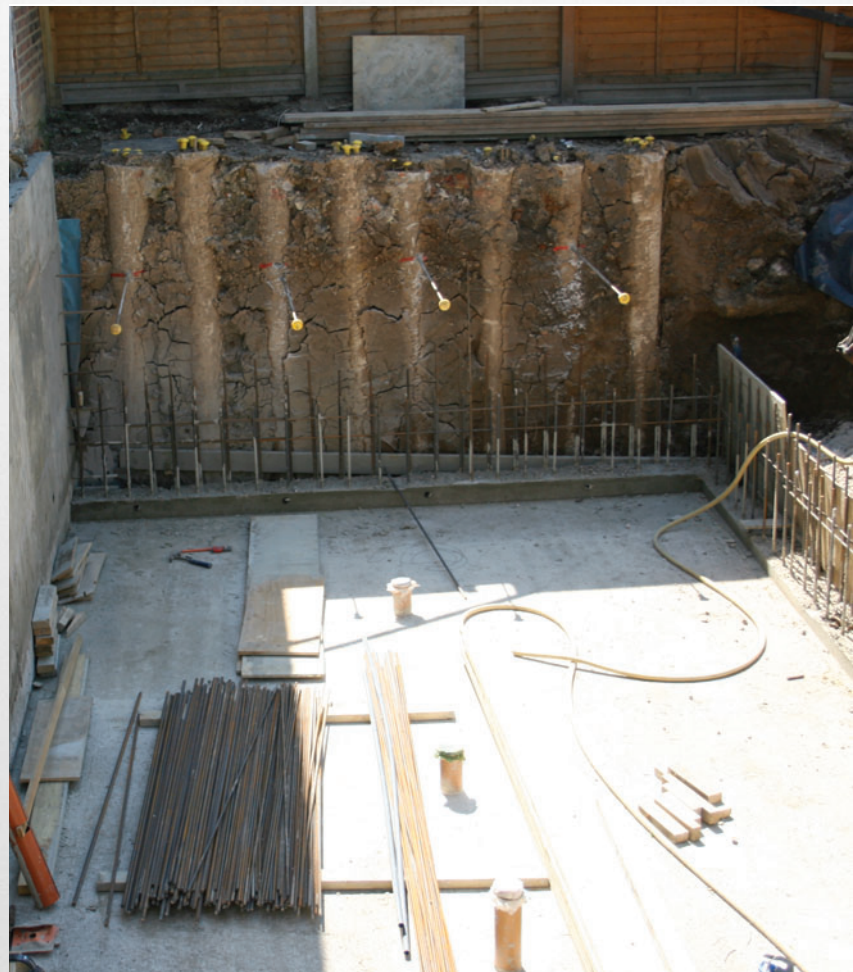
Underpinning Basement
