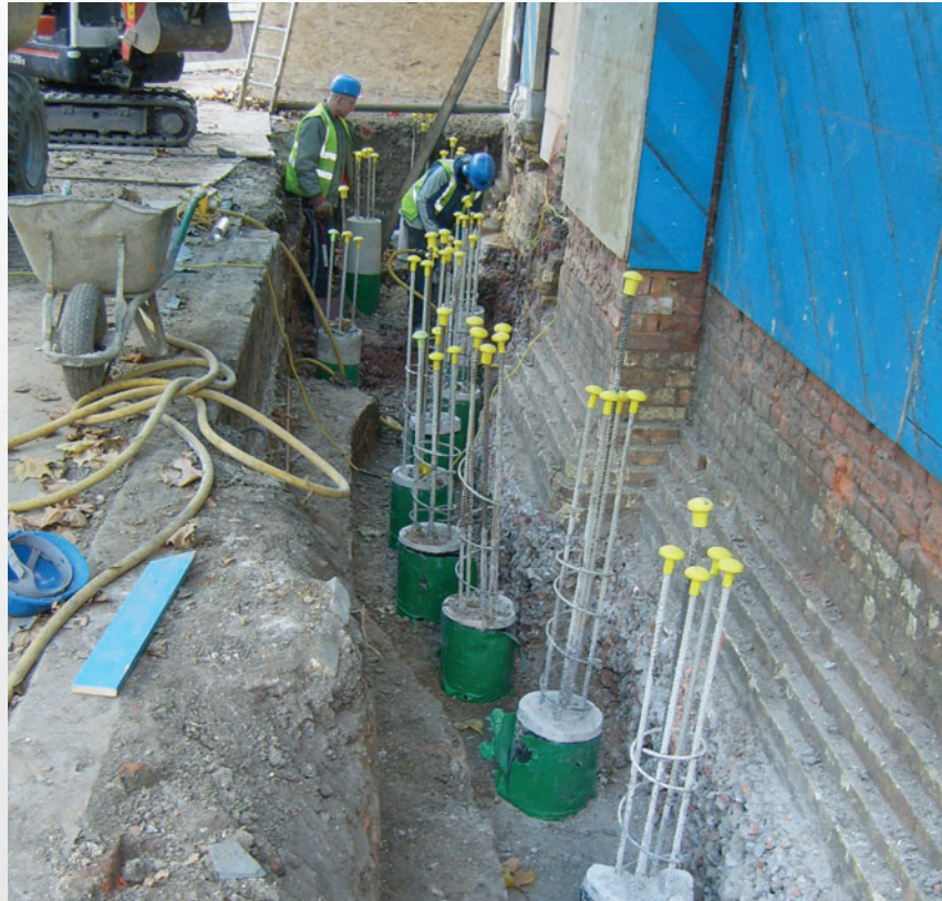
Installed augered piles
