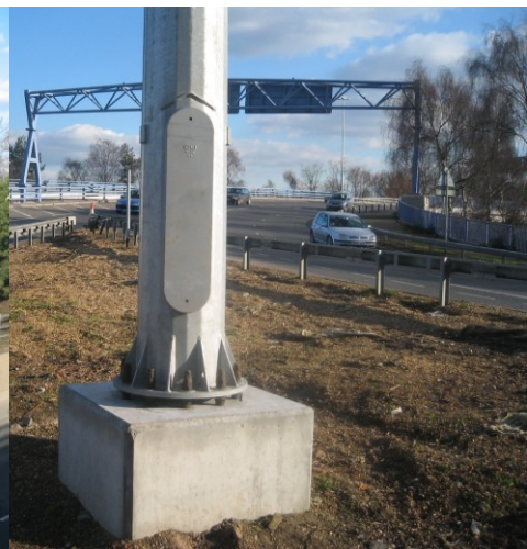
Column installed between the main carriageway and the slip road on the inner city ring road.
