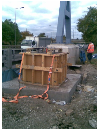
A column base being cast next to the A52 post-piling.
