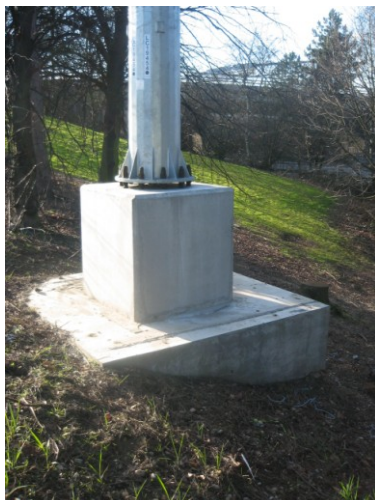
High mast piles, base and plinth installed on a slope.
