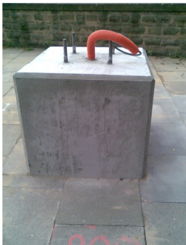
A cast plinth ready for the lighting column to be attached.
